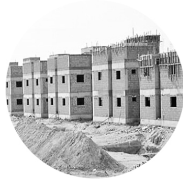
Residential developments under construction without spatial link to their immediate context.
