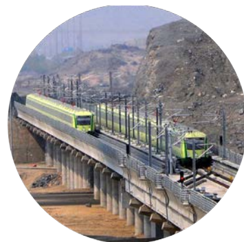
The existing metro line running in the Al-Mashaer area
