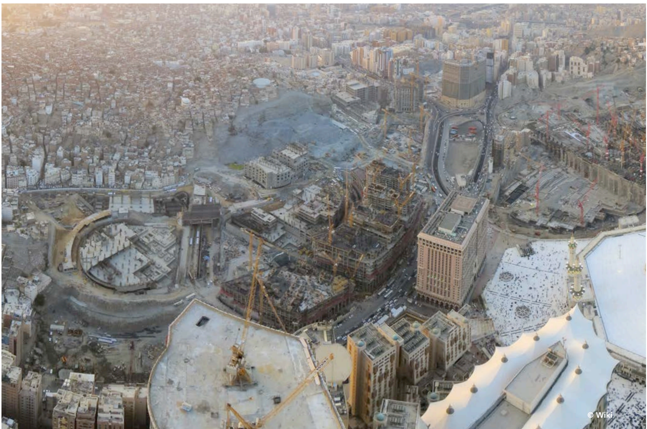
View of construction sites and unplanned settlements in Makkah
